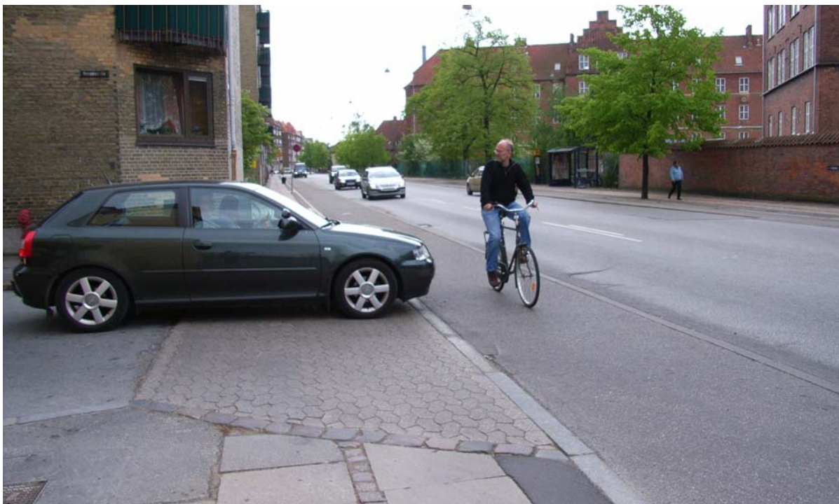
Side road junction with elevated cycle track crossover
