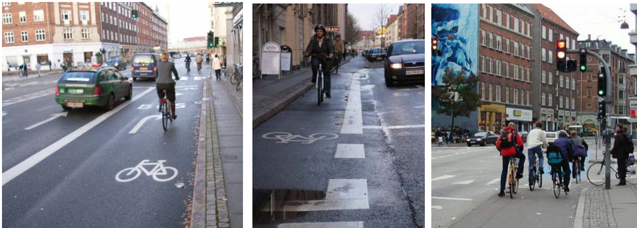
Shortened cycle track extended into a right turn-lane (left foto), a shortened cycle track extended into a narrow lane (middle) and an advanced cycle track with a blue cycle crossing and a pre-green light for cyclists (right).
