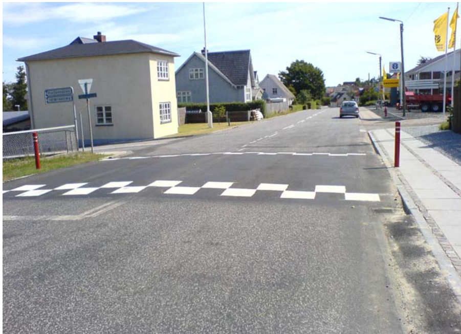
Figure 6 Traffic calming at school route in Frejlev.
