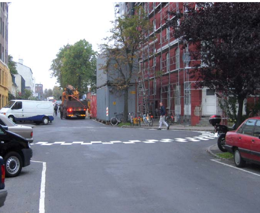
Untraditional use of 'dome hump' to ensure safety at a small junction in a residential area.
