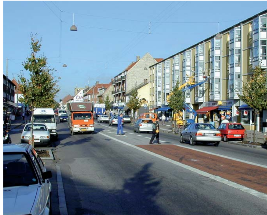
A road redesigned from four lanes to two lanes with a mid-section island, ensuring the safety of crossing pedestrians.
